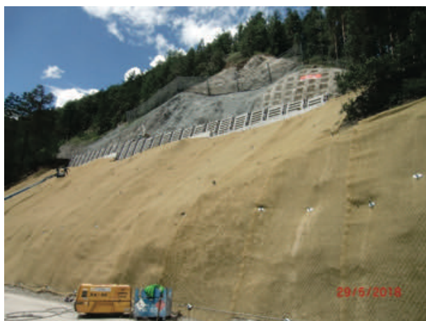
Figure 15 Final works underway at the Serfauserstrasse, with a highlight on the greening mat along the bottom part of the road.
