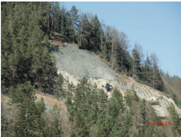
Figure 9 View of the unstable slope at Ladiserstrasse, where the first part of anchoring and mesh deployment is completed, allowing secure works underneath to be completed.
